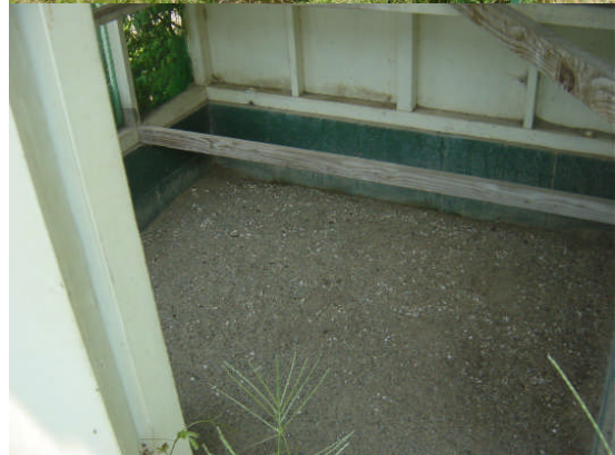
(Photograph 3) Naraha North elementary school
